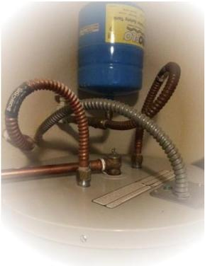
Periodically check the water supply lines and the valves for any sign of water. Mineral deposits around the connections might also indicate imminent failure. Rust is an obvious sign of a slow water leak. That includes the expansion tank connected to the water heater. If the water heater fails suddenly (cracks or leaks) turn off the water closing the valve located right above the tank.
