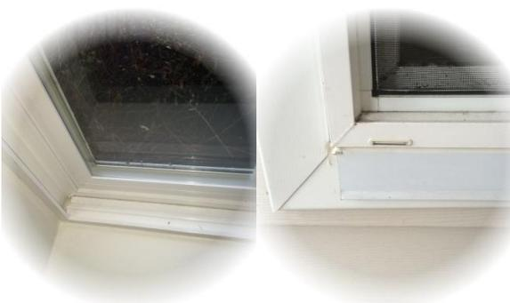
Some residents reported water standing in the window track (left picture). This happens rarely due to condensation on the window. Most of the time is just rain pushed by the wind in between the fixed and the sliding windows. All this water should drain outside. But if the "weep hole" (right picture) is closed or clogged the water will not drain. You can open and/or clean the weep hole by removing the screen from inside.
