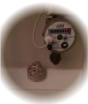
If any sudden leak or flood happens (i.e. pipe burst etc.), turn off the water in your entire apartment. You can do that by closing the valve located under one of your bathroom sinks, next to the water meter (see picture). By doing this you minimize tremendously the extent of the damage. It is extremely important to know the location of this valve. Even five minutes sooner make a huge difference when a major water leak happens.
