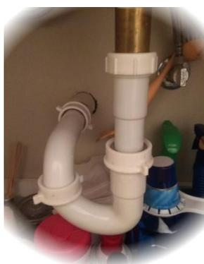
Do not clutter the space under the sink making it inaccessible. Inspect this space every month, at least, to make sure there are no leaks. Hitting the drain assembly multiple times can make the couplings and gaskets to come loose. Also check the supply lines and the valves.
