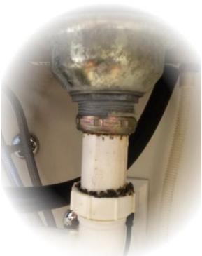
Over the years owners called to report the kitchen sink leaking. Half of the time it turned out to be the metal coupling that connects the drain assembly (P-trap) to the sink itself (see small metal coupling in the picture). This coupling is not the right size (too small) and it tends to come loose over the years. I recommend replacing it with a PVC one, which has more threads to grab on.
