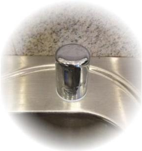
If you see water coming out of the air gap, it means the dishwasher's drain line is clogged. This is caused by dirty dishes not pre-washed prior to putting them in the dishwasher. The air gap can clog too but most of time is just the hose. In the next picture I will show you how to unclog it.
