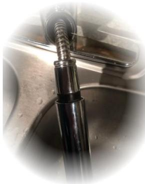
A lot of small leaks are caused by the sink faucet. The part that you pull out tends to unscrew over time and if not noticed, it will leak under the sink without even seeing it. You just need to hand tighten it. As an extra step you can add Teflon tape on the threads before screwing it back in. Check it every once in a while to make sure it didn't come loose.
