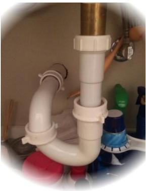
Do not clutter the space under the sink making it inaccessible. Inspect this space every month, at least, to make sure there are no leaks. Water under the sink can be the result of multiple issues. Do not ignore it. Check the supply lines and the valves first.
