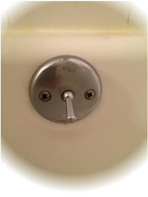
The overflow gasket is extremely important because it can cause a lot of damage without being noticed immediately. In the past we had cases where the damages exceeded \$10,000. And all this because of a part that costs \$3 (in store at Ace Hardware or at Home Depot online) and can be installed in 5 minutes. I suggest replacing it every year, especially if you are taking baths. In order to replace it you need to remove the cover completely but it is held in place by only 2 screws.
