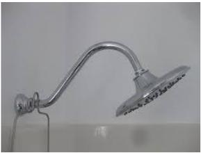
Make sure that the shower head is not leaking or spraying water on the walls above. If you replace it make sure the new one is tight, seal it with Teflon tape and do not over tighten it. When you do it hold the extension in place, not to come loose inside the wall. Oversized shower heads tend to spray a lot more water around increasing the chance of getting water on the walls.
