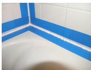
Caulking around the bath tub is essential. Make sure that is intact and not separated from the wall. If it is missing in some areas you might end up with a lot of damage in your unit and not only. If it needs to be replaced, scrape it all off and start fresh. You can use painter's tape (see picture) to help you make it look professional. I recommend re-caulking the bath tubs every year with silicone caulking.
