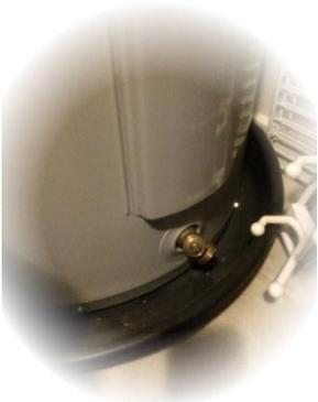
Inspect the tray under the heater for any sign of water. If you see even a small amount that means the heater started cracking at the bottom. Five minutes of your time periodically spent checking could save you days of headaches and quite a bit of money. Also part of the maintenance of your water heater should be the annual flushing of the tank. Contact me for more details on how to do that.
