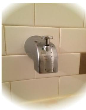
Pay attention to the tub spout. If you see water coming from under it when you pull the switch, it means that the built-in gasket is damaged and the spout needs to be replaced. If you don't do that the water might "shoot" back into the wall where you can't see it and cause a lot of damage. To remove the spout you need an Allen key (Hex key) and can be tricky sometimes. When you install the new one do not over tighten it because you might perforate the copper line.
