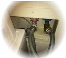
Check the water supply lines and the valves of the washing machine for any water leaks, look behind the machine periodically. Also make sure that the drain hose is inserted properly into the drain and secured with a zip tie or something similar.
