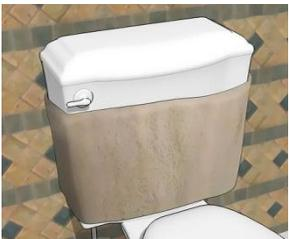
Another common problem in the bathrooms is water around the toilet. Rarely the culprit is a supply line or the tank. Most of the time this is the result of the condensation on the tank and bowl. For more information about it read this article: <http://www.wikihow.com/Stop-Toilet-Tank-Sweating> If you have vinyl flooring in your bathrooms and see dark spots on it that might be caused by a faulty wax ring or some other kind of water leak. Investigate it immediately.
